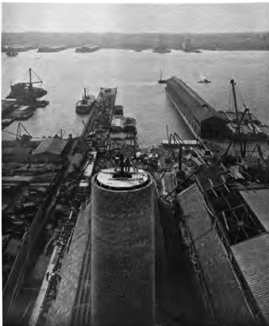
VIEW FROM TOP OF CHIMNEY SHOWING WATER FRONTAGE — POWER HOUSE
